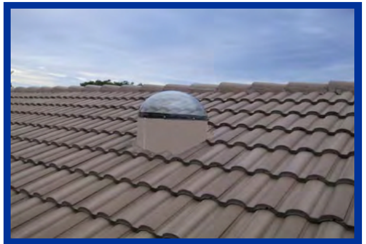
Tile roof application.
