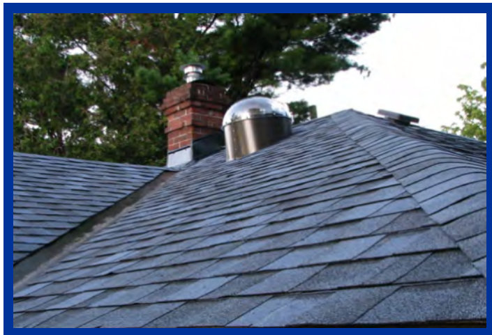
Shingle roof application.
